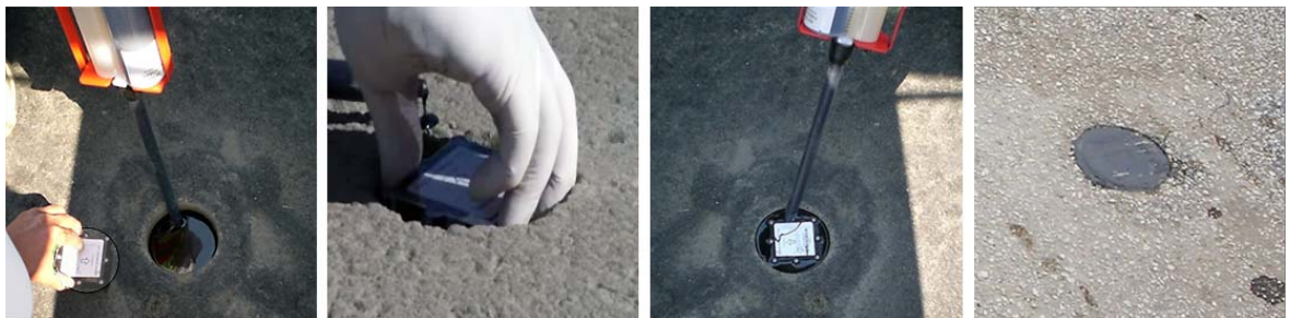
Figure 4.2 – Epoxying Sensor Into Hole
