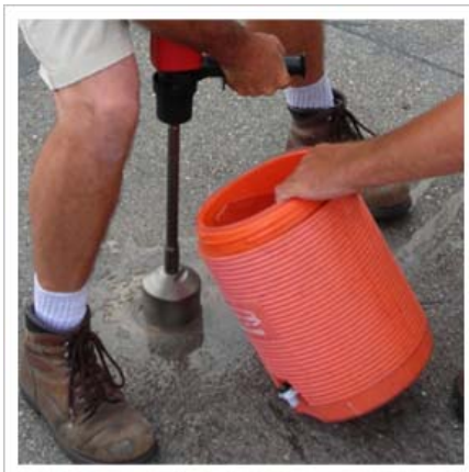
Figure 3.9 – Coring Sensor Hole
