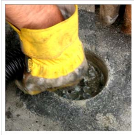
Figure 3.10 – Clearing Sensor Hole
