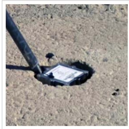
Figures 3.13, 3.14– Filling Hole With Epoxy
