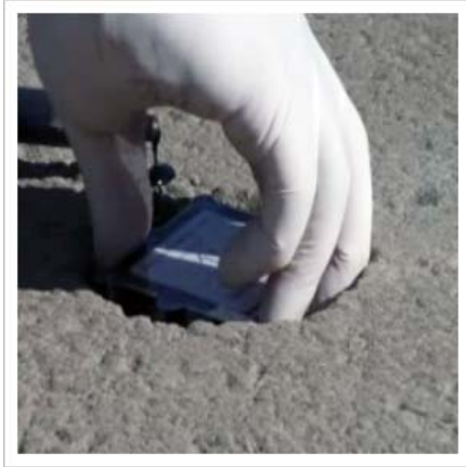
Figure 3.12 – Placing the Sensor in Road
