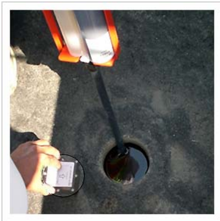
Figure 3.11 – First Epoxy Application
