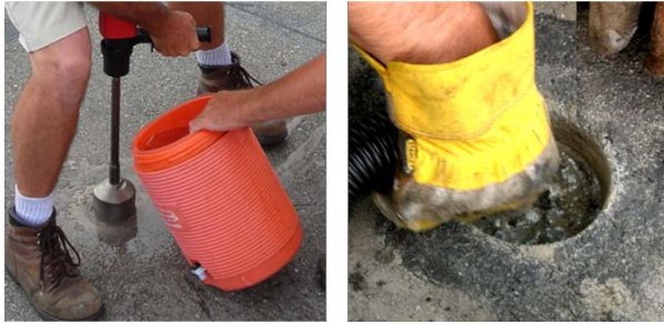
Figure 4.1 – Coring and Clearing a Sensor Hole
