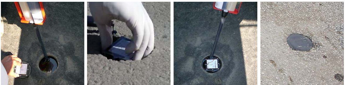
Figure 4.2 – Epoxying Sensor Into Hole
